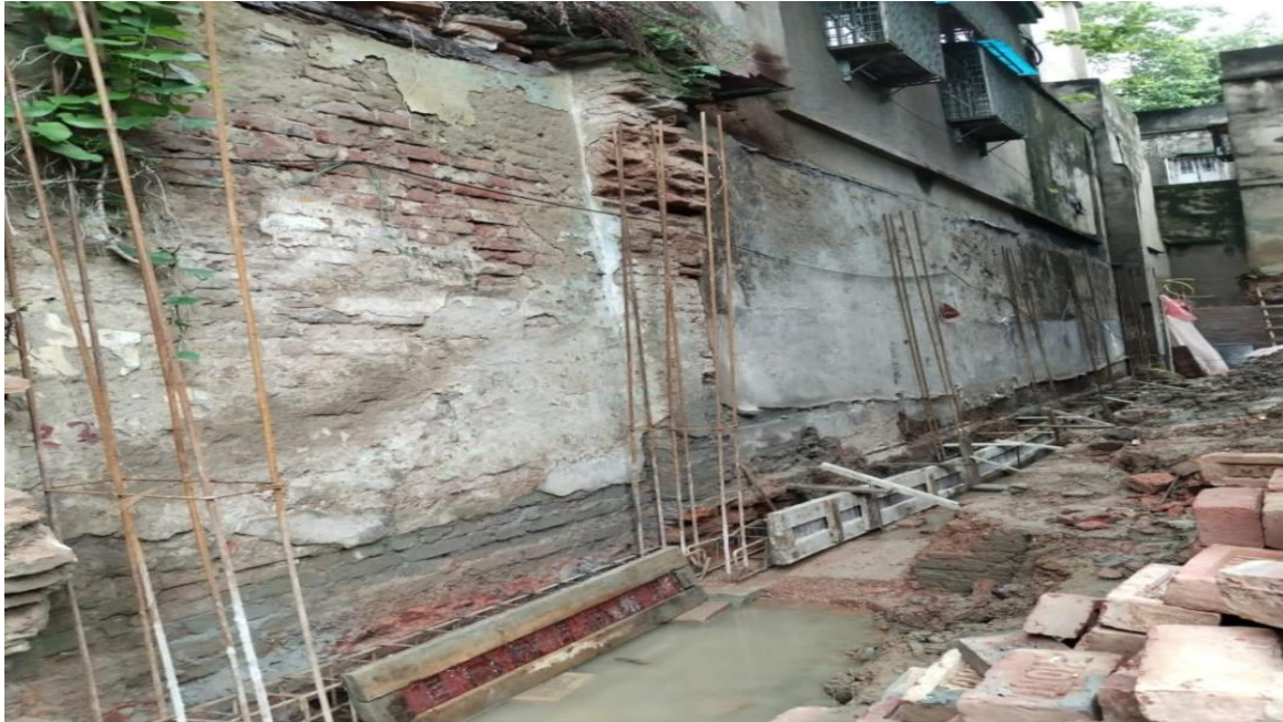
South side boundary work going on
